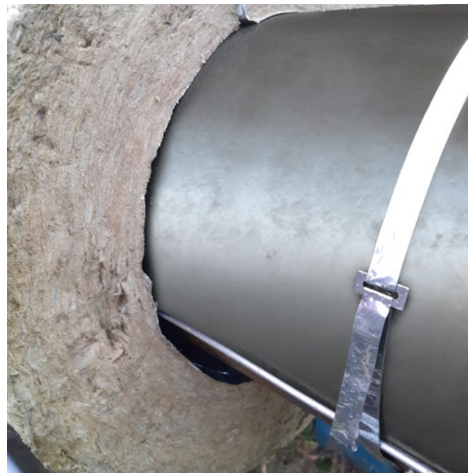
↑ INNOVATIVE METHOD USING PAROC PIPE SECTION ALUFOAT WR 100 INS
