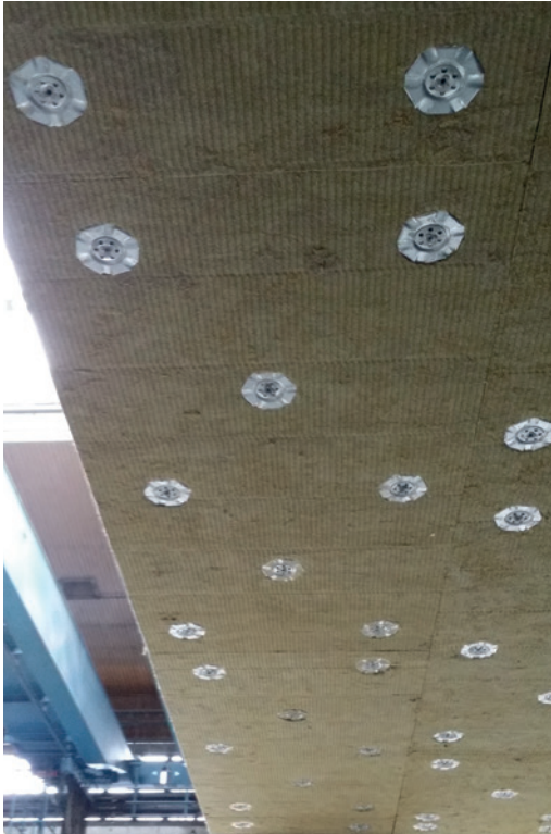
Fire protected concrete slab.
