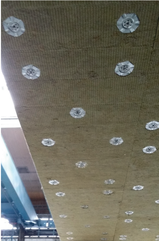
Fire protected concrete slab.
